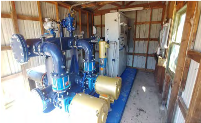
Stafford Country Club, Batavia, NY. and their MCI - 1000 GPM, Vertical Turbine Pump Station with 2- 60 hp pumps installed in 2019
